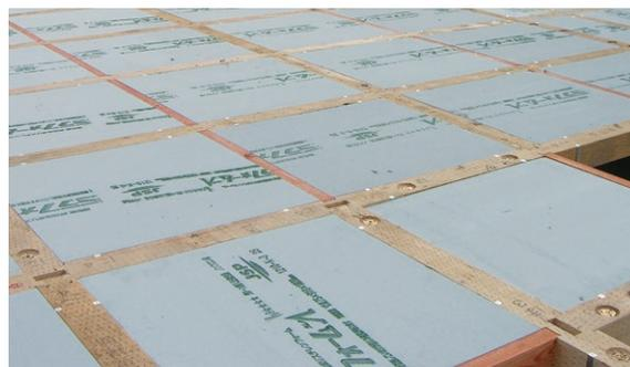
Pre-cut thermal insulation material MIRAFOAM (lambda)
